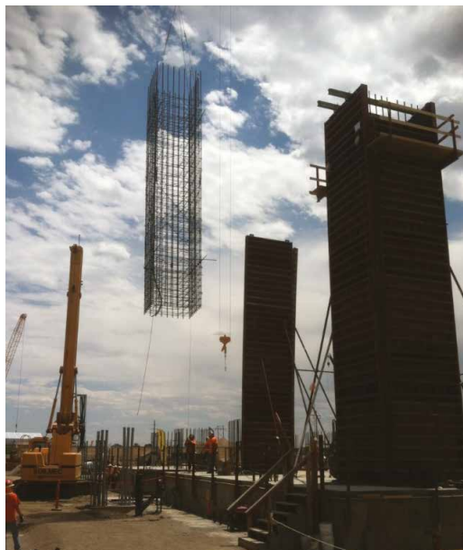
Fig. 11-3. Column rebar cage being flown into place
