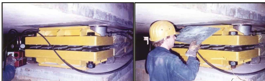
Fig. 10-20. Height adjustment is possible, if required Source: Courtesy of GERB Vibration Control Systems; reproduced with permission.
