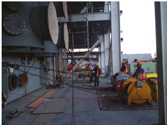
Fig. 11-7. Condenser installation utilizing air winches and heavy equipment rollers (2)
