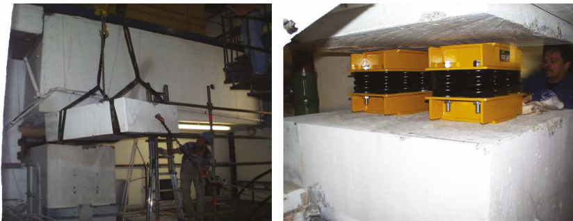
Fig. 10-16. Typical steps for retrofit of a TG tabletop
